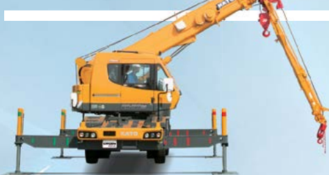
Hoist the auxiliary rope and swing out the Jib.
